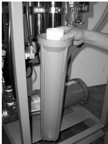
Illustration 13 - Sediment Prefilter Cartridge
